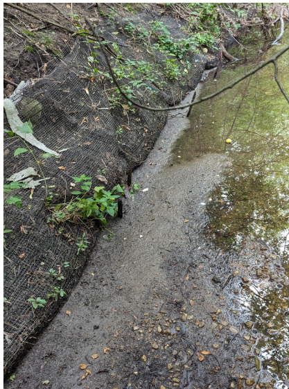
Left: Reach 3 plastic netting as lost soil from behind the netting and the bank shows erosion above the netting. Sediment has accumulated at the bottom of the channel slope. Right: Reach 3 soil bags along outer bend of channel with concrete ajacks toe.
