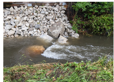
↑ J-hook structure under high flows after a stabilization project in Urbana, Illinois.
